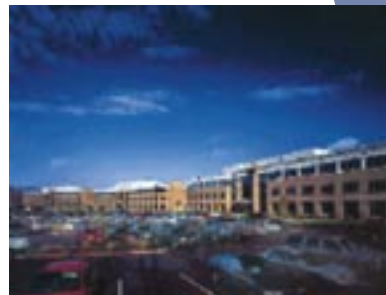
Orion Office Buildings
